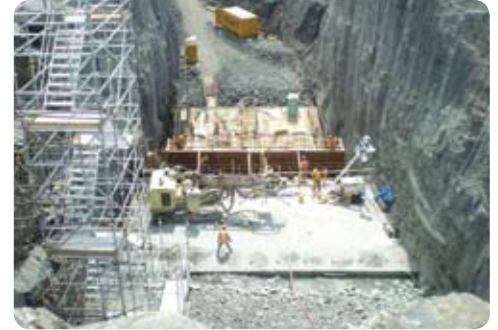
Redevelopment work on the Hound Chute generating station’s powerhouse.
